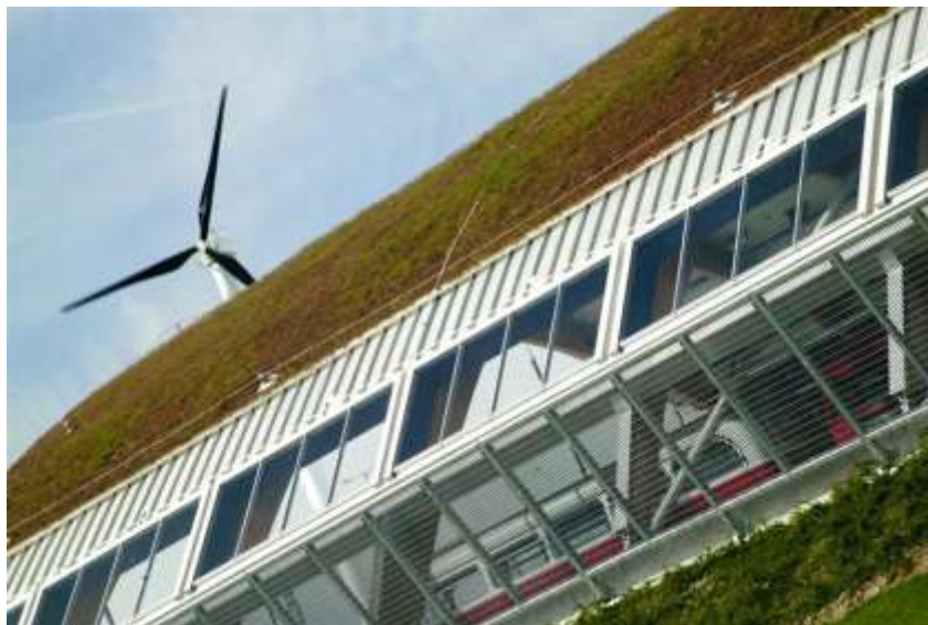
West Ham Bus Garage. Image courtesy of Kalzip Limited
